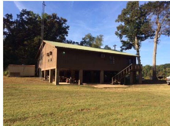
Lodge with dry storage under lodge
